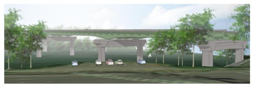
The new Abernethy Bridge, shown here with new strengthened columns, will be able to withstand a major earthquake
